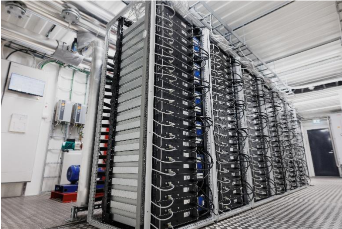
Bitcoin data center with custom-built high-end servers for efficient heat and Bitcoin generation
